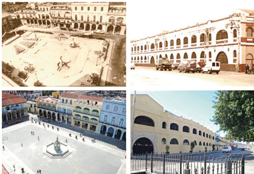
Fig. 18.2 Restoration works in Old Havana. Note: Old Square (left) and Old Warehouses of San José (right). (Source: Havana Historian Office. Master Plan (OHCH 2015))
